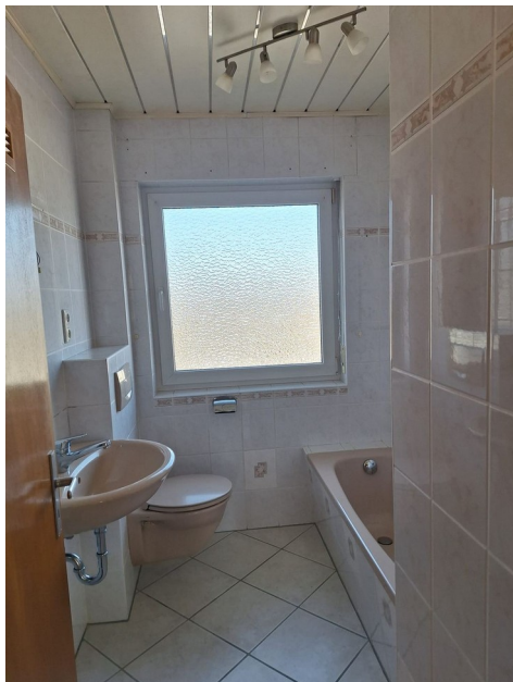
Bad (OG) – Ist-Zustand
