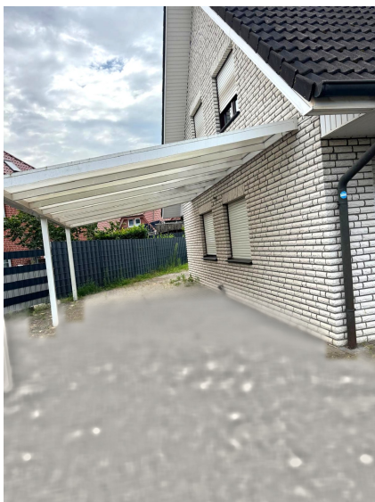
Carport (ca. 17 m 2 )
