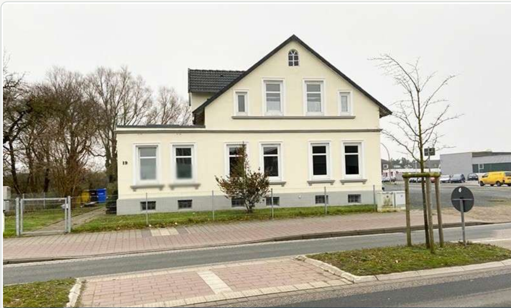
Two-unit residential building on Brockeswalder Chaussee
