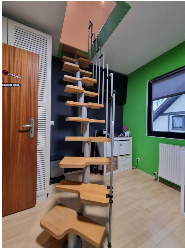
Raumspartreppe in Spitzboden
