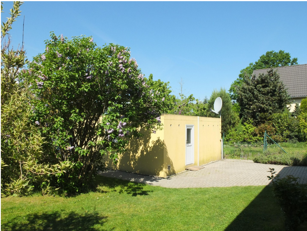
Blick zur Garage
