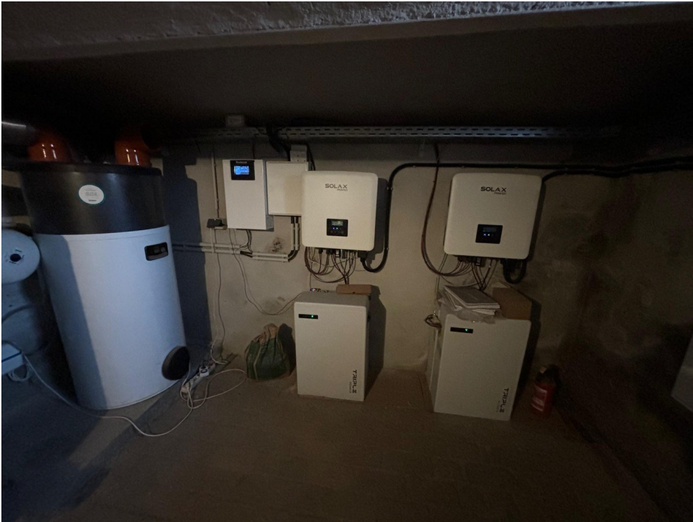
Akku System PV-Anlage
