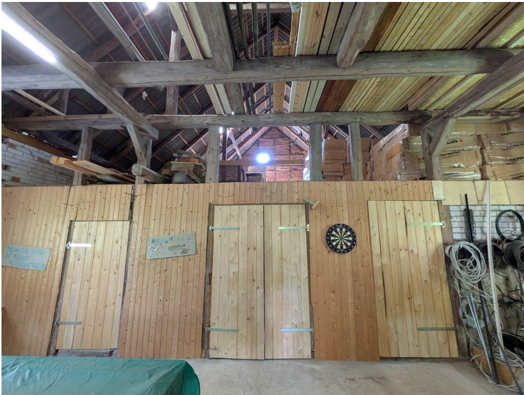
Blick in Scheune - 2. Boden
