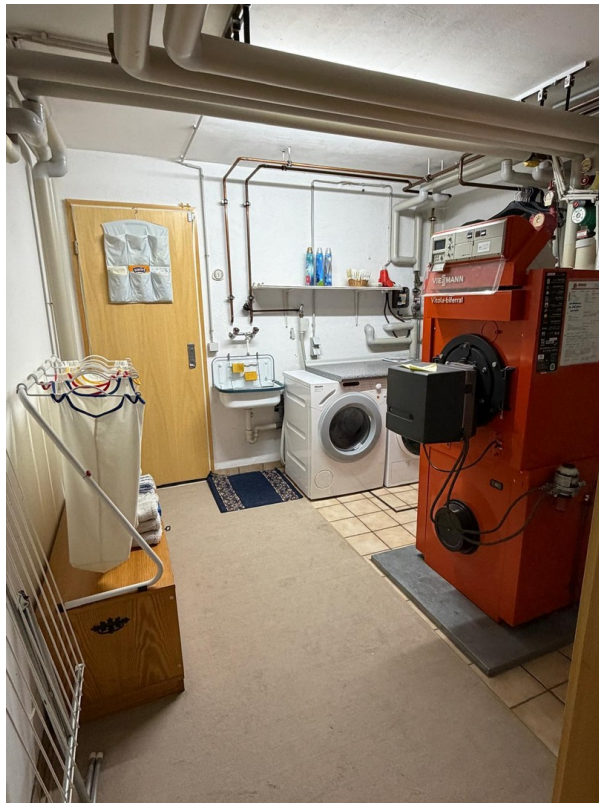
Heating and Washing Basement
