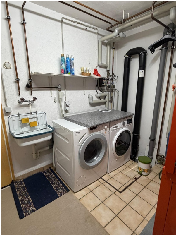
Heating and Washing room
