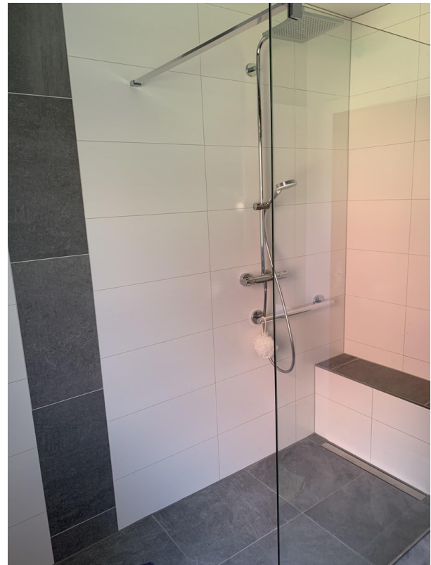
Bad / Walk in Dusche EG
