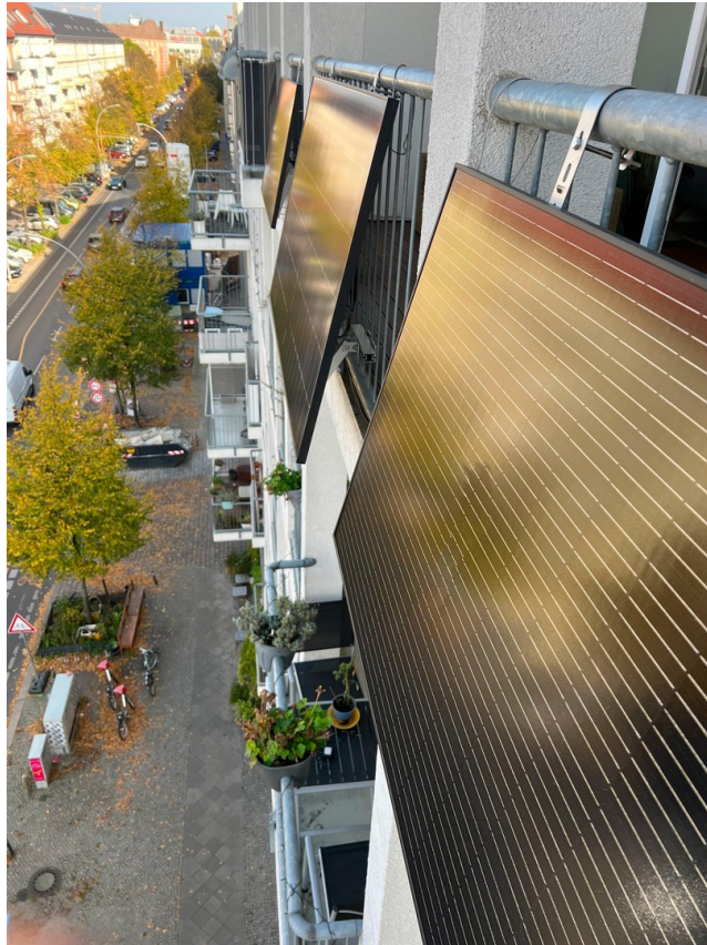
Solar Power System
