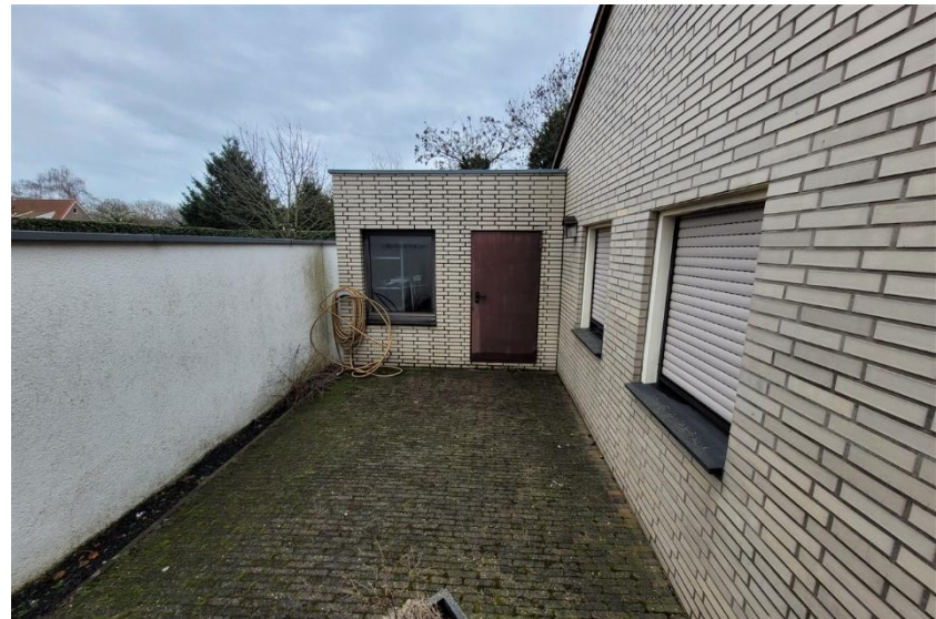
Foto A 8: Abstellraum - links
