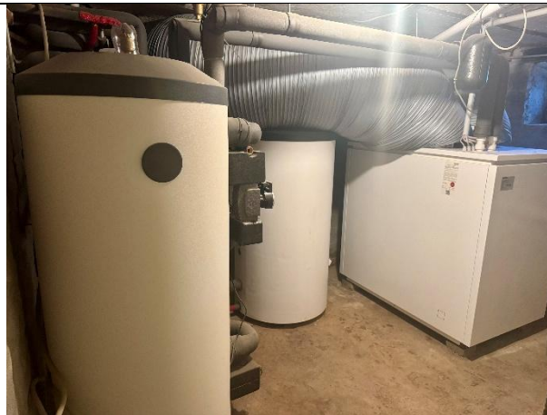
Internal heat pump Stiebel Eltron WPL 19 installed in 2022
